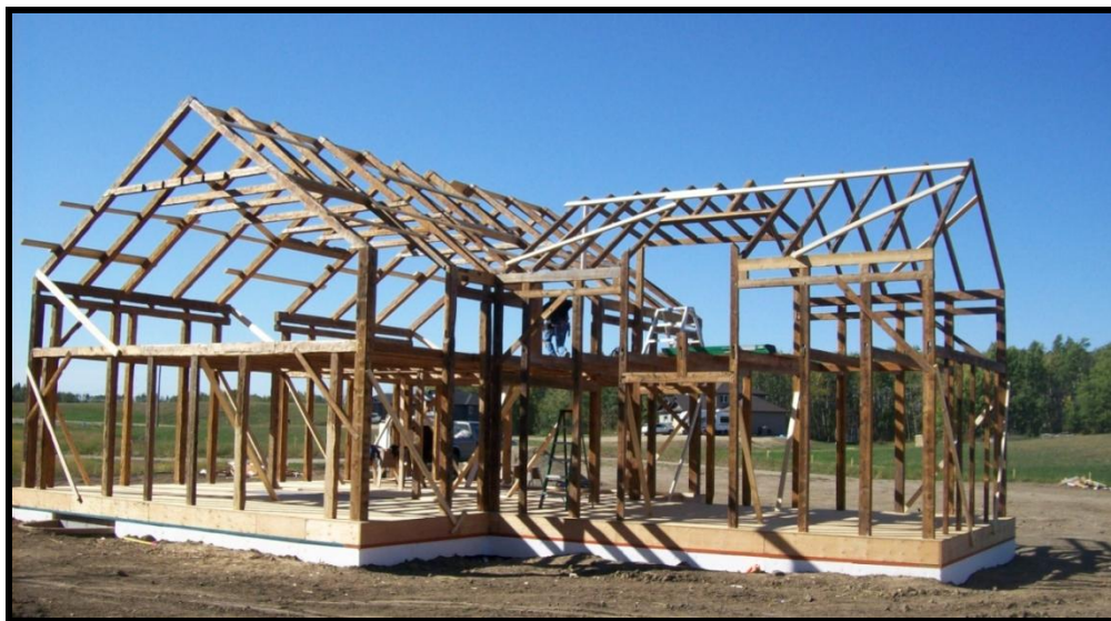
Modified and Re-Installed
