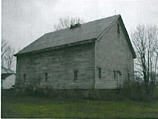
1) Corner of building showing the gable-end and one long side
