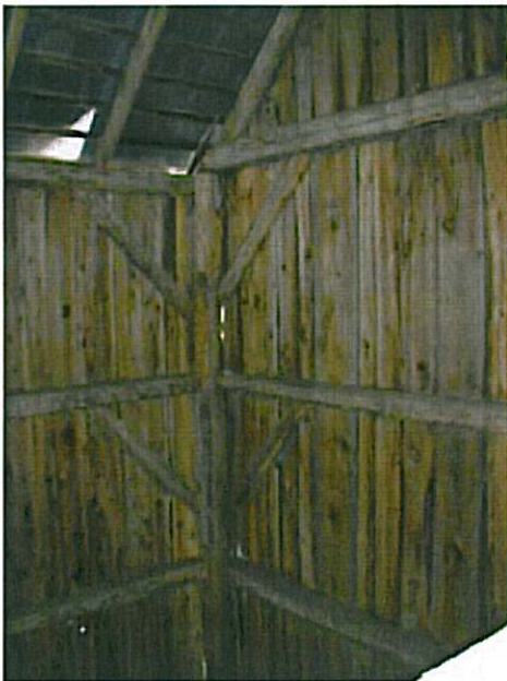
6) Corner post with braces and other connecting beams
