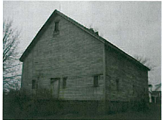
2) Opposite corner of building showing the other gable-end and long side
