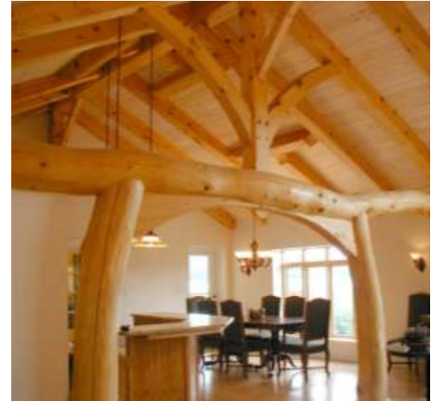
King Post with Crown bracing
