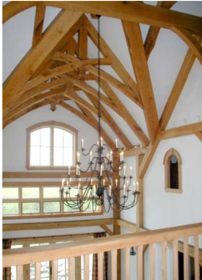
Scissor Trusses with King Posts
