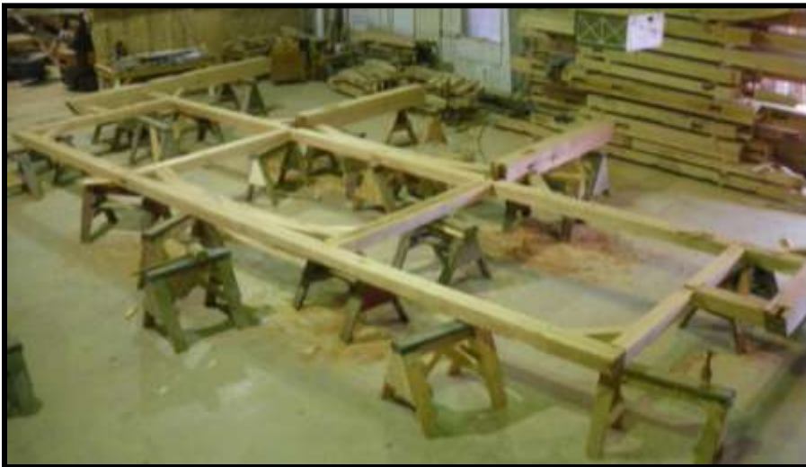
Timber Section being pre-fitted
