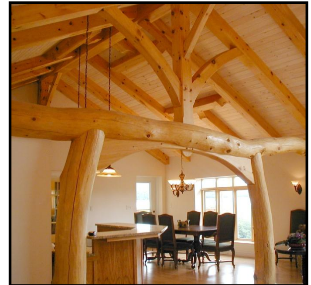
King Post with Crown bracing
