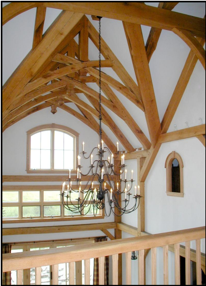
Scissor Trusses with King Posts
